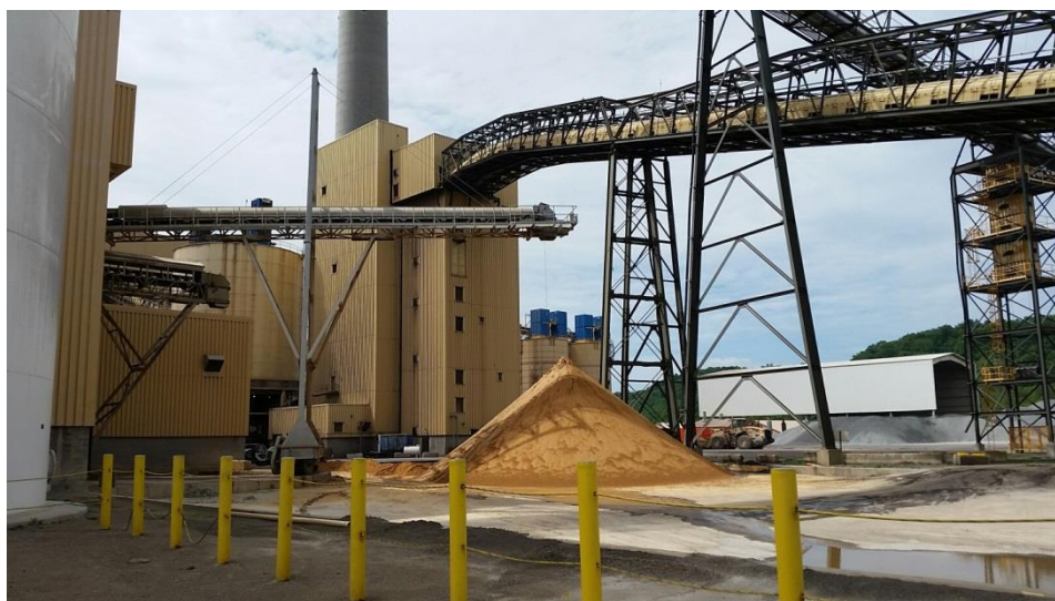
Figure 3-6: Gypsum Pile and Load Out Operations
