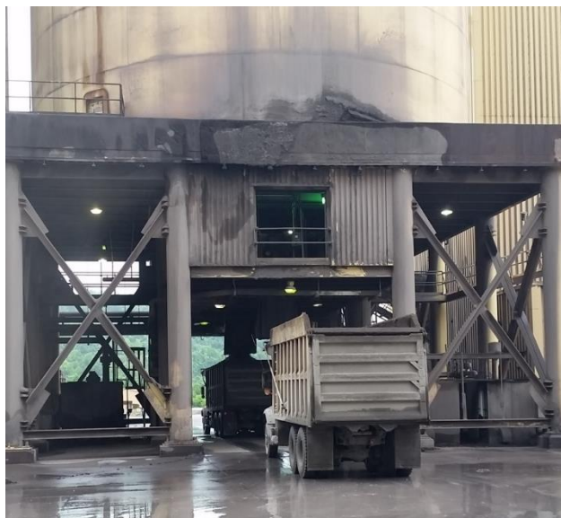
Figure 3-3: U3 Fly Ash Truck Loading Operation
