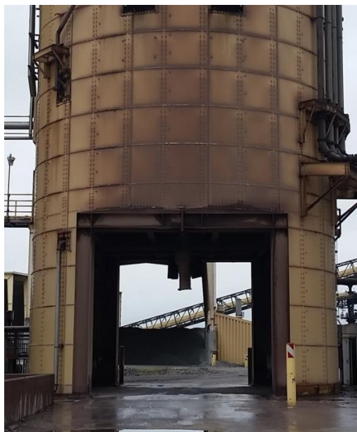
Figure 3-4: U4 Bed Ash Loading Operation
