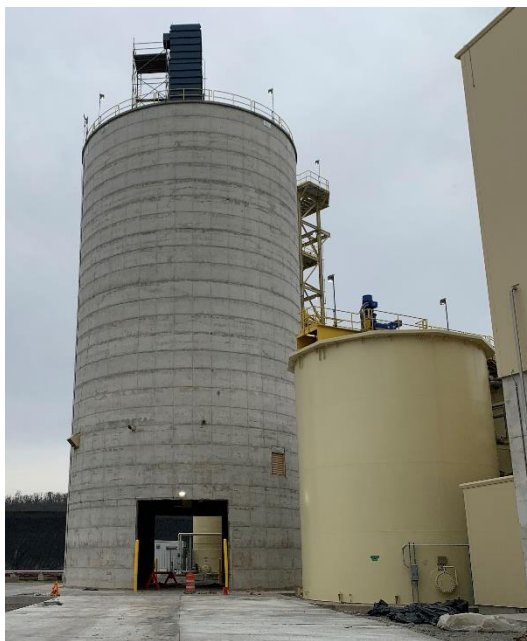
Figure 3-11: New U1/U2 Fly Ash Silo Loading Operation
