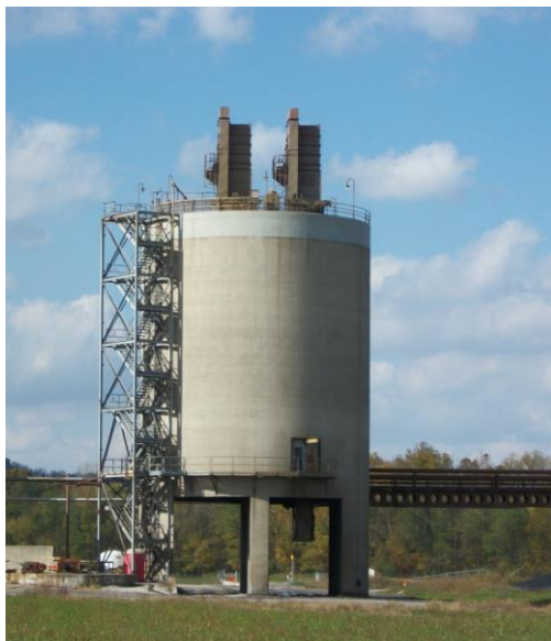
Figure 3-1: Spurlock U1&U2 Fly Ash Load Out
