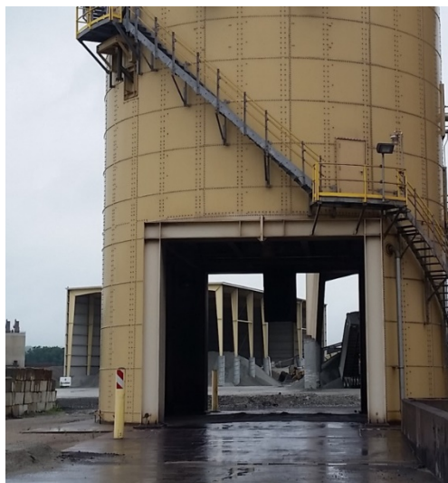
Figure 3-5: U4 Fly Ash Loading Operation
