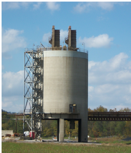
Figure 3-1: Spurlock U1&U2 Fly Ash Load Out
