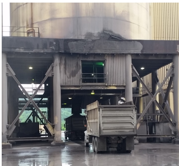
Figure 3-3: U3 Fly Ash Truck Loading Operation
