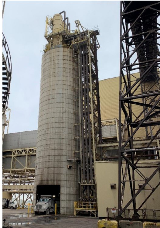
Figure 3-10: U1/U2 Bottom Ash Loading Operation
