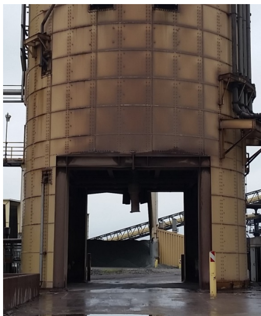
Figure 3-4: U4 Bed Ash Loading Operation
