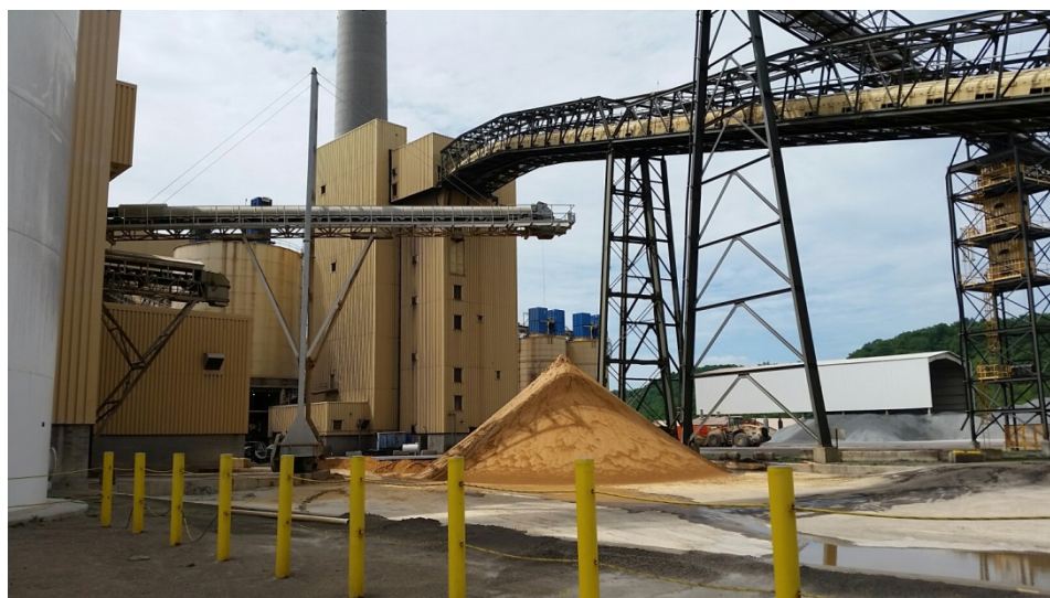
Figure 3-6: Gypsum Pile and Load Out Operations
