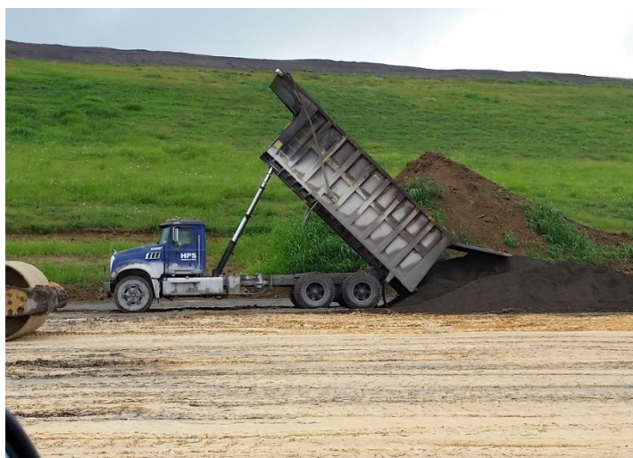
Figure 3-8: Truck Unloading at Landfill
