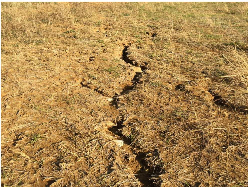
Photograph Number: IMG-7542 Description: Final cover lack of vegetation
