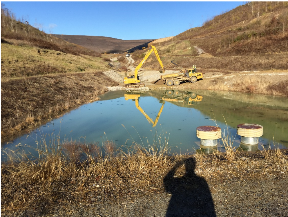
Photograph Number: IMG-7482 Description: Pond 1, looking west. Cleanout activities taking place.
