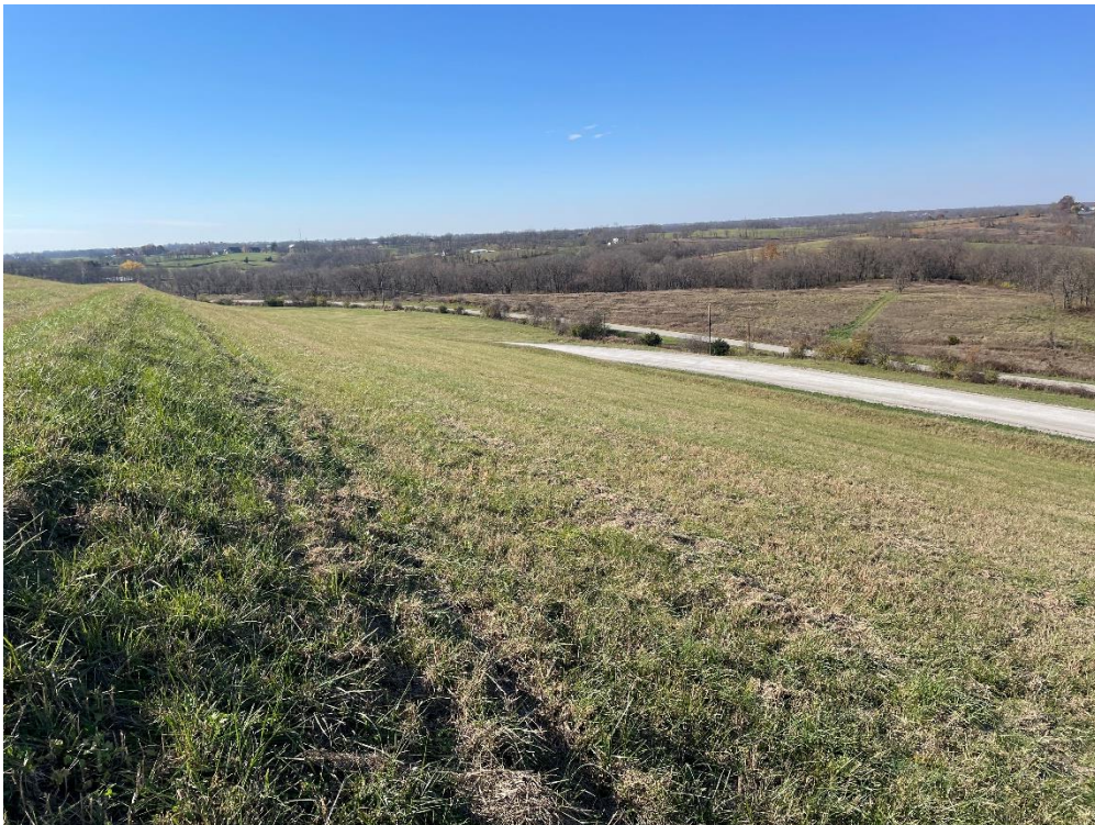
Photograph Number: IMG-2501 Description: Final cap – West slope
