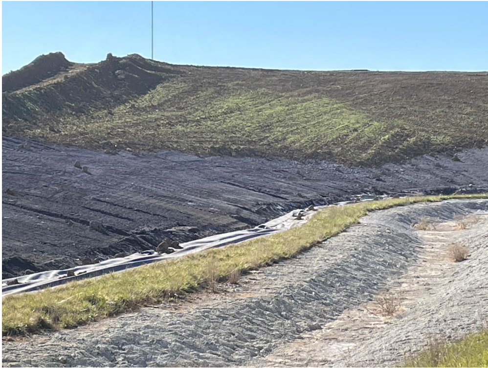
Photograph Number: IMG-2562 Description: Area C Phase 5 – North perimeter ditch
