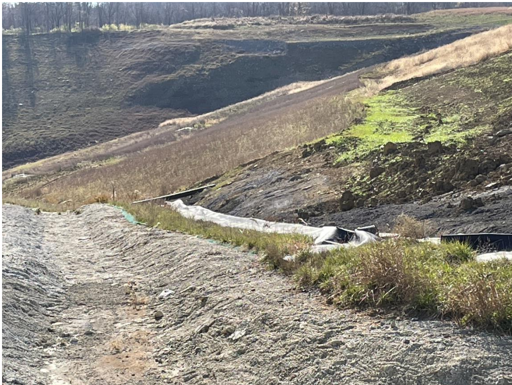
Photograph Number: IMG-2563 Description: Area C Phase 4 and 5 – NE perimeter ditch
