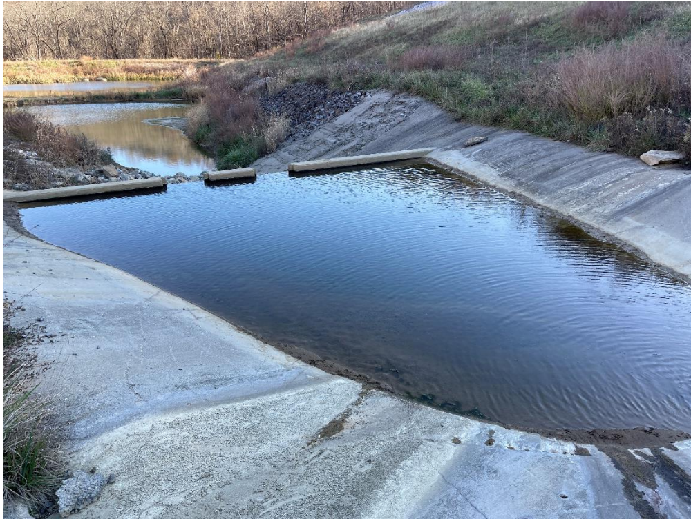
Photograph Number: IMG-2618 Description: Pond 1 – Clean out concrete sediment trap
