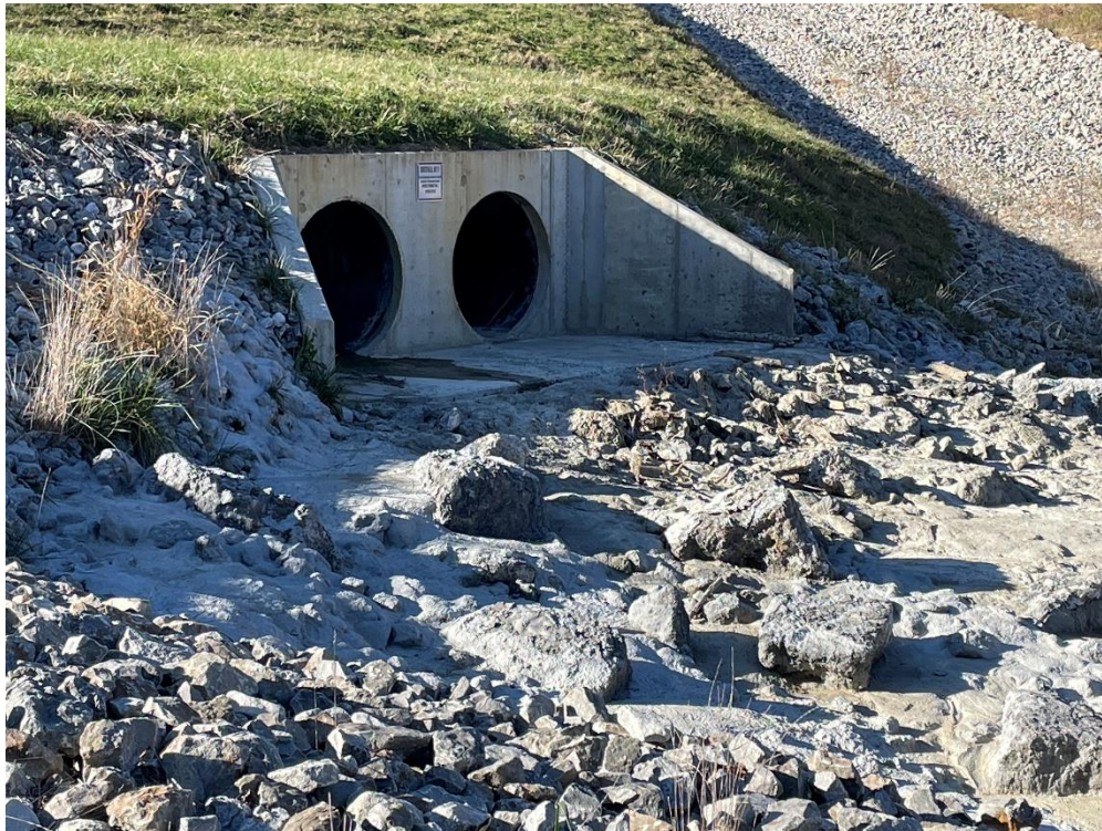
Photograph Number: IMG-2609 Description: Pond 2A Discharge
