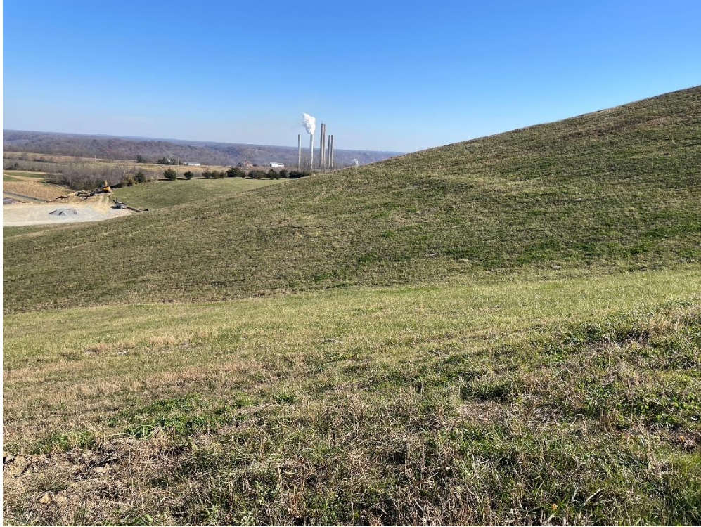
Photograph Number: IMG-2499 Description: Final cap – NW Slope
