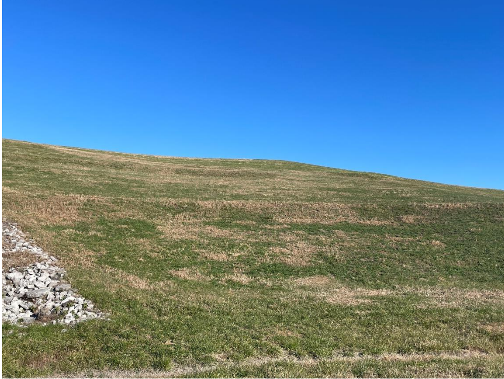
Photograph Number: IMG-2469 Description: Final Cap – South Slope
