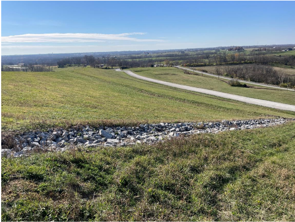
Photograph Number: IMG-2489 Description: Final cap – SW slope
