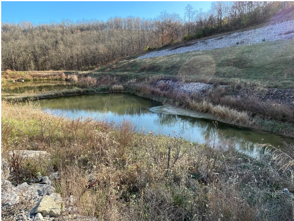
Photograph Number: IMG-2617 Description: Pond 1 Upper chamber – Clean out sediment
