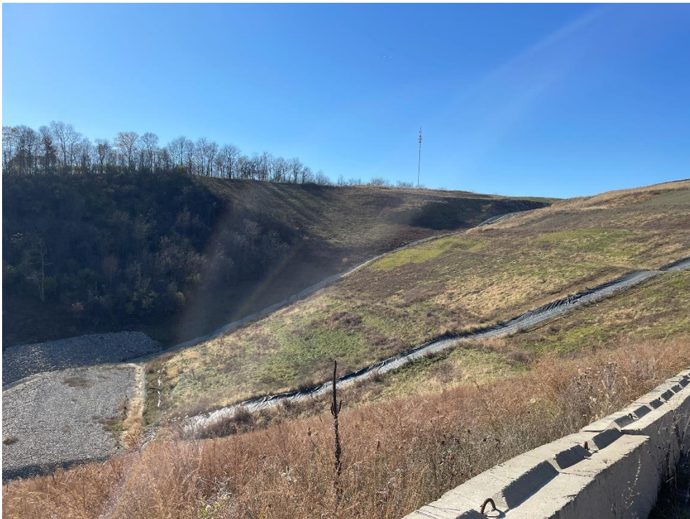
Photograph Number: IMG-2565 Description: East Slope – Area C Phase 4 & 5
