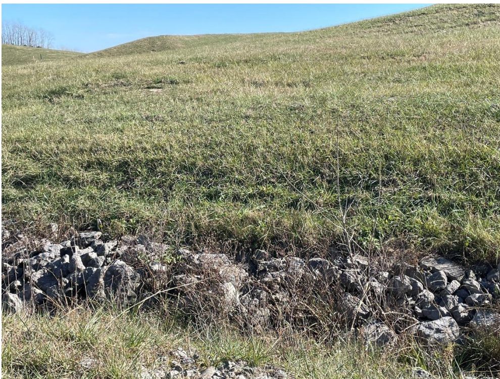
Photograph Number: IMG-2542 Description: West final cap, NW – Remove woody vegetation growth
