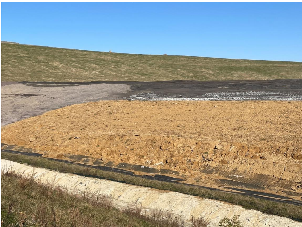
Photograph Number: IMG-2472 Description: Area C, Phase 5 – South perimeter ditch
