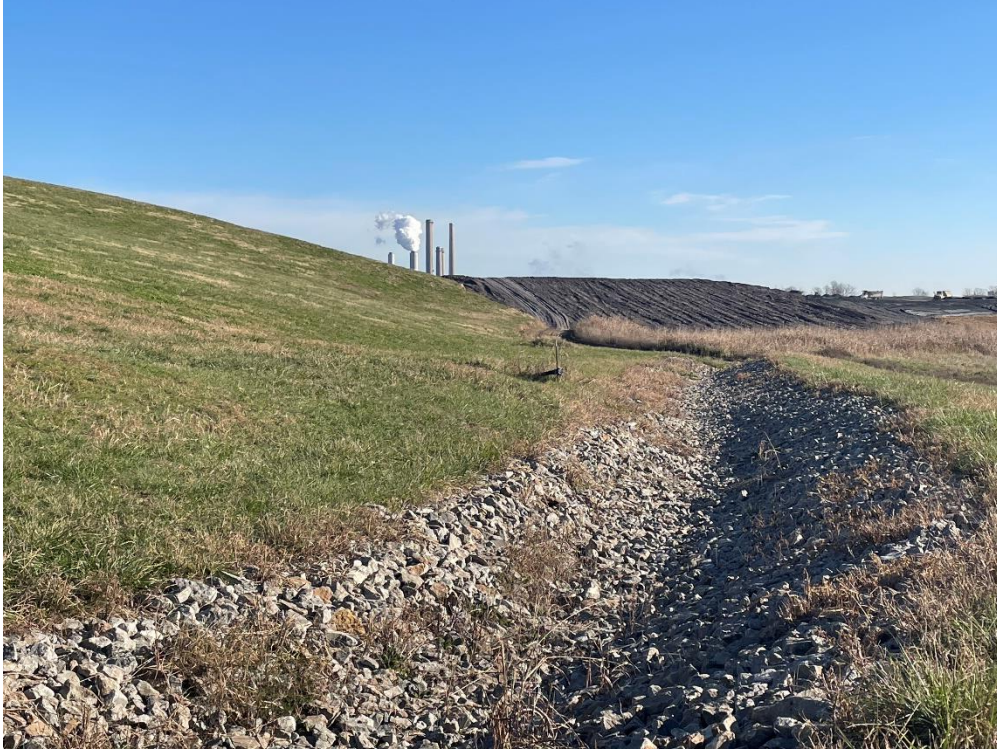
Photograph Number: IMG-2471 Description: Final cap – South perimeter ditch
