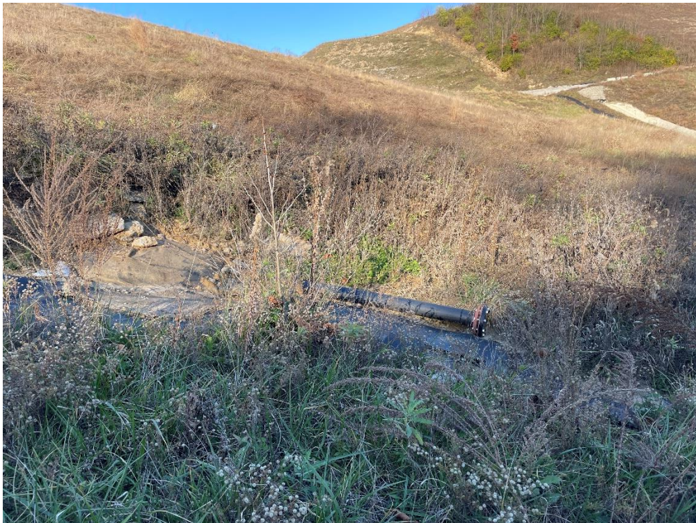
Photograph Number: IMG-2623 Description: Area C Phase 4, SE – Woody vegetation growth
